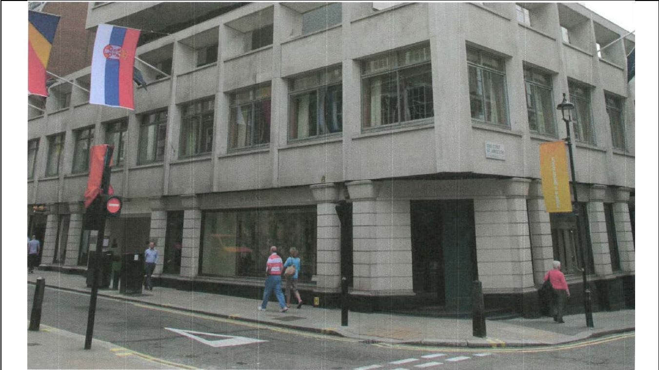
Existing Jermyn Street
