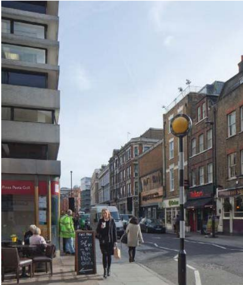
26-29 Drury Lane (above) & 12 Dryden Street (below)
