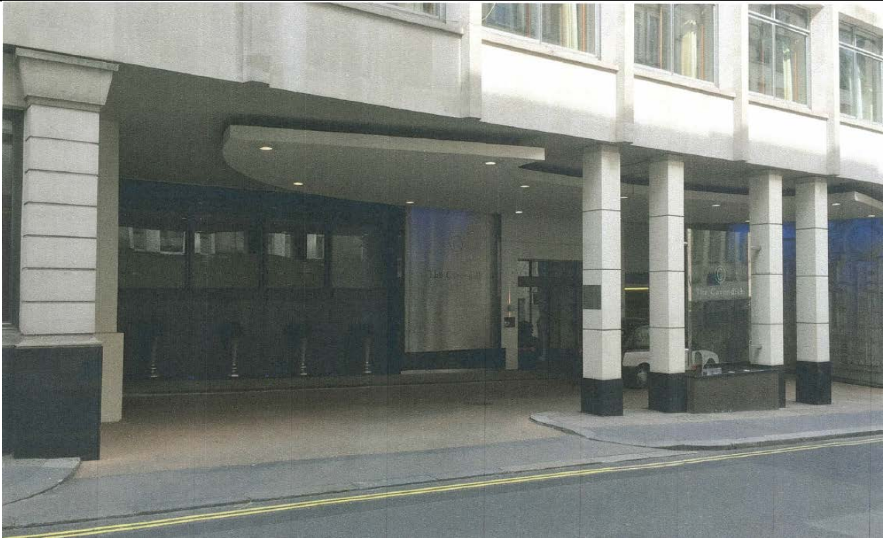
Existing Duke Street St. James's
