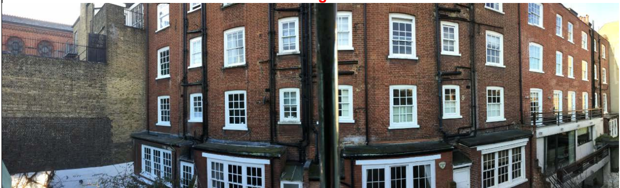
View from rear of 32 St Petersburg Mews looking at rear elevation of 18 St Petersburg Place and neighbours
