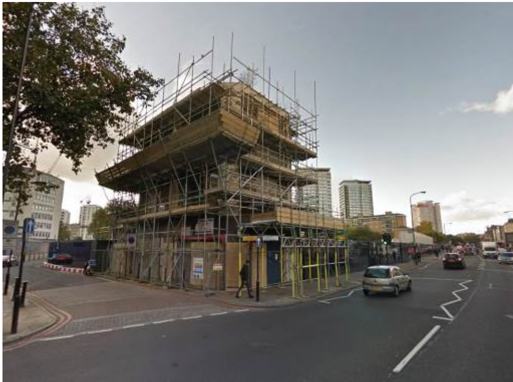
View of application site at Church Street/Newcastle Place junction
